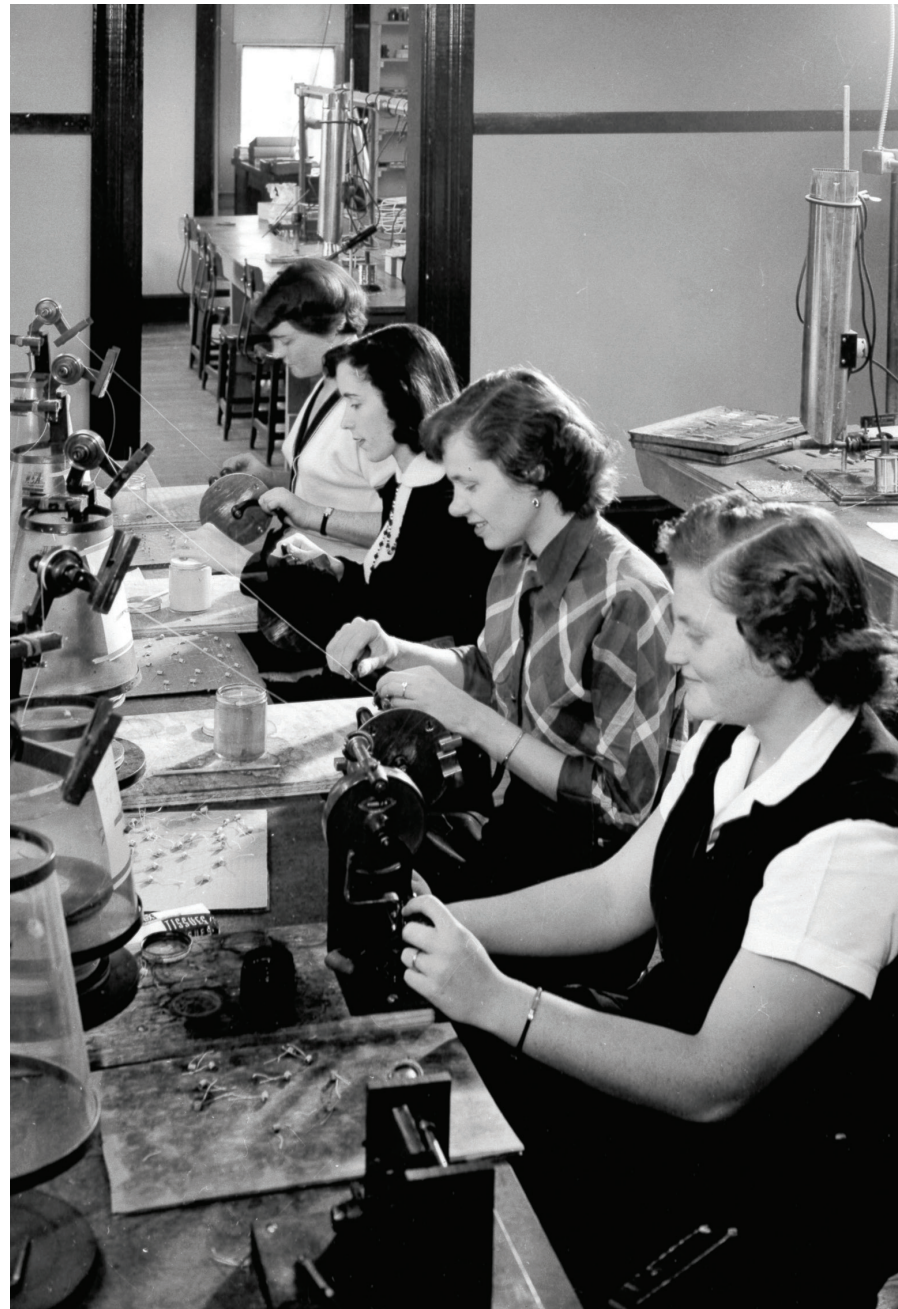
Coil winding rooms in first Sturgis factory
