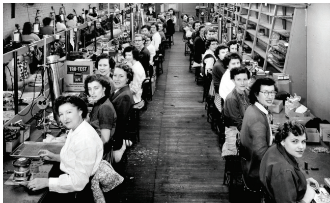
Main assembly room floor in Sturgis, KY manufacturing facility
