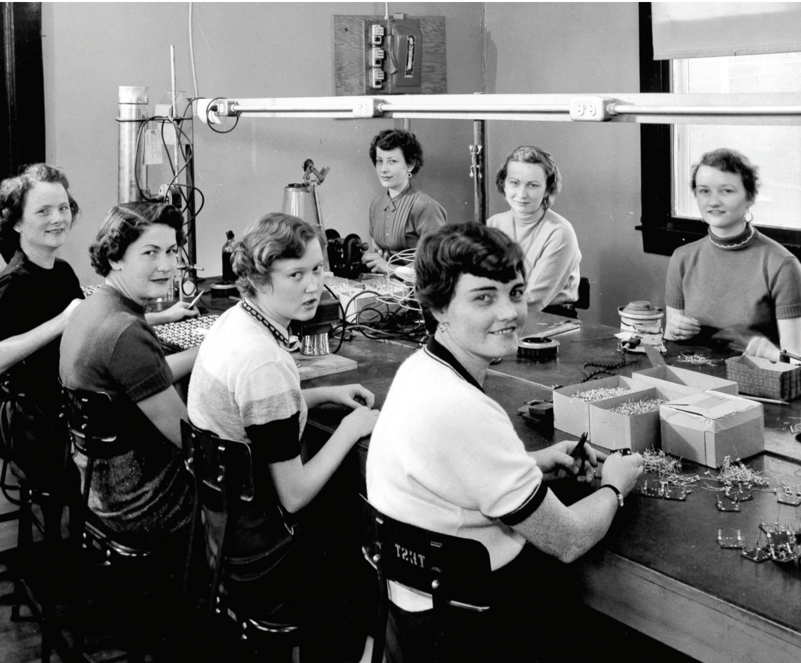
Coil winding rooms in first Sturgis factory
